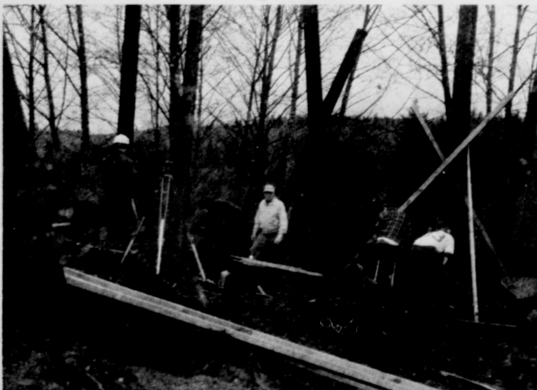
WORK PROGRESS last weekend on the Garden Pavilion at the Oral Hull Park for the Blind. The building which will be used by the Touch and Grow—Garden Club for the blind is being constructed by members of the Clackamas and Multnomah District Garden Clubs. This past
