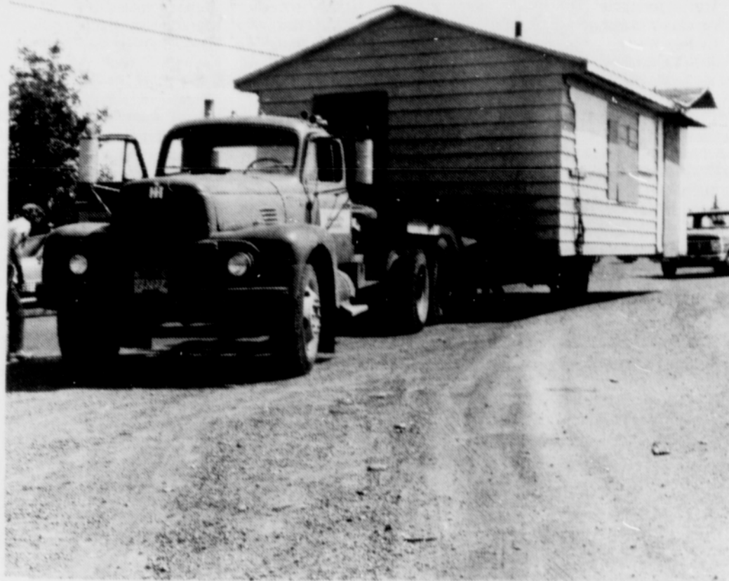
A MOVING house or a moving van? This house created a minor traffic jam in downtown Boring last week as it moved to its new site.
