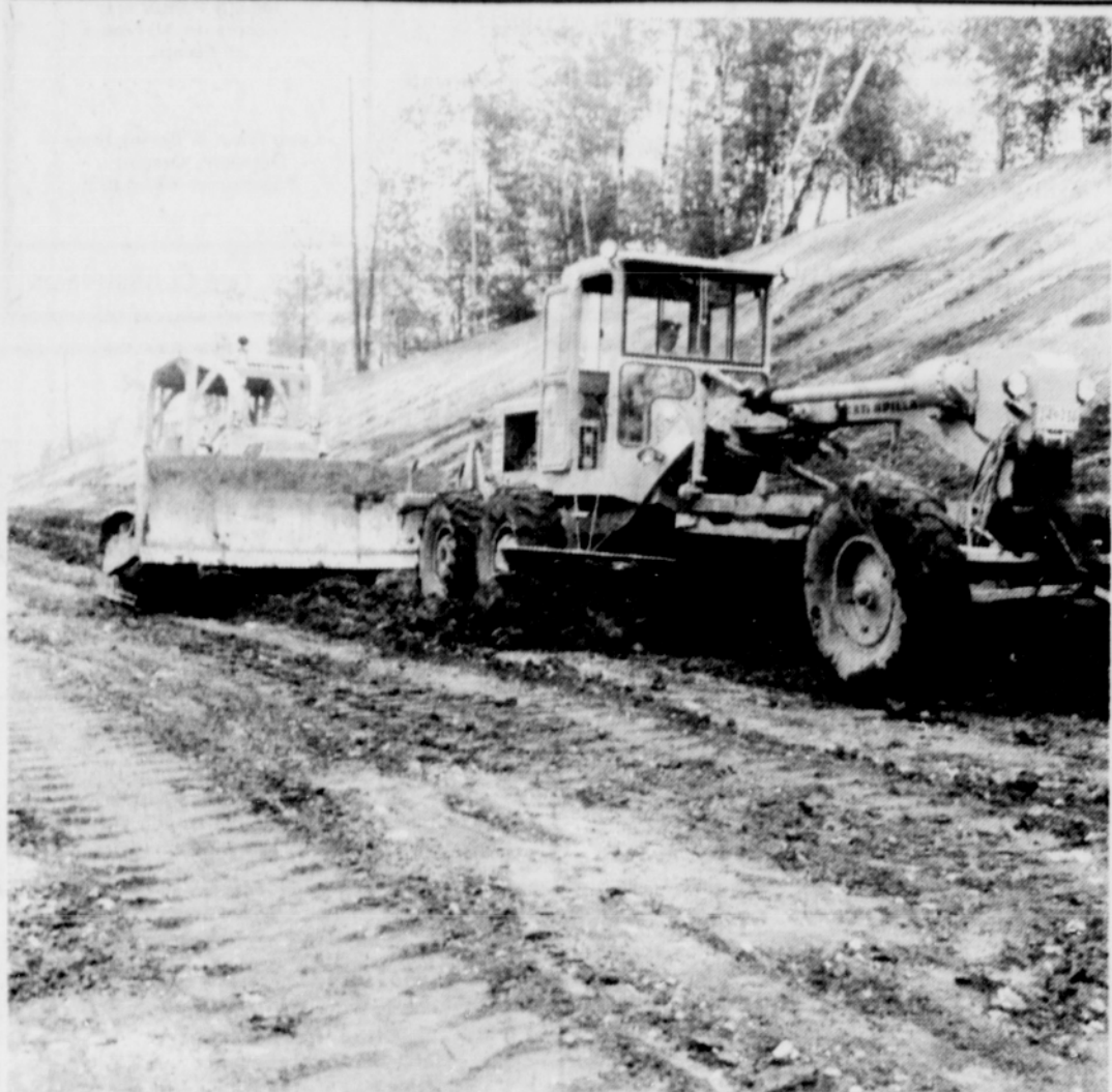
SOME WORK has begun on Highway 26 between Aldercreek and Brightwood. The road is expected to be completed by this
