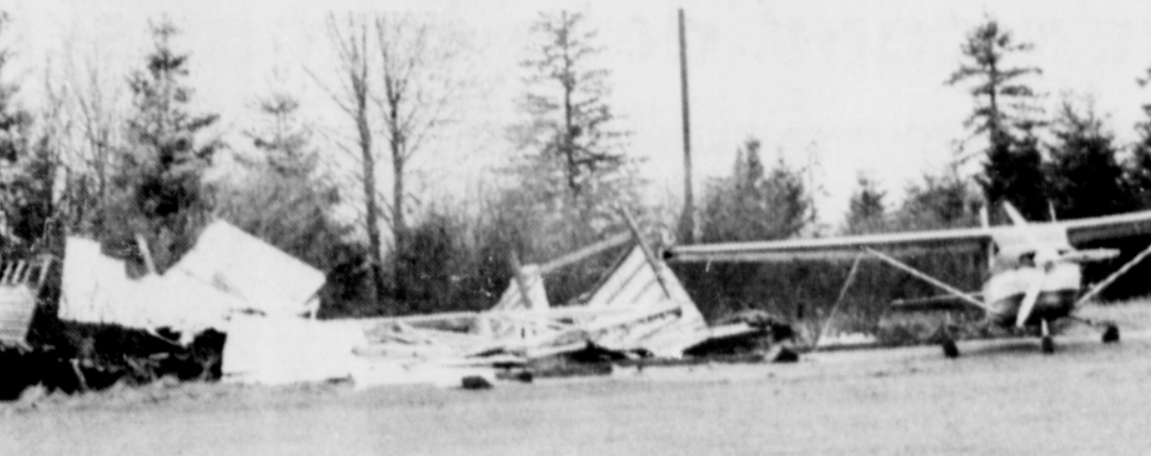
STRONG WINDS last Wednesday demolished an airplane hangar at the George Cushman residence, Rt. 1, Box 780, Boring, but left the plane (above) virtually intact. Cushman, for whom the hangar had been built just six weeks ago, placed the
