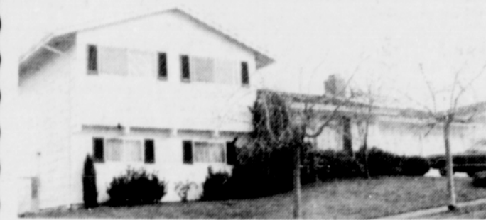
4 BEDROOM TRI LEVEL —3 bedrooms up, 1 down, 2 baths, fireplace, wall to wall carpet, drapes, range, party room with wet bar, attached garage, covered patio, above ground swimming pool with deck, cyclone fenced, nicely landscaped yard, fine neighborhood. Only $28,500.
