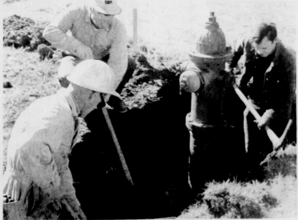
THERE IS more work being done on Scenic Ave. in Sandy than adding a new curb. Everything in its way is being moved back a few feet such as this fire hydrant.
