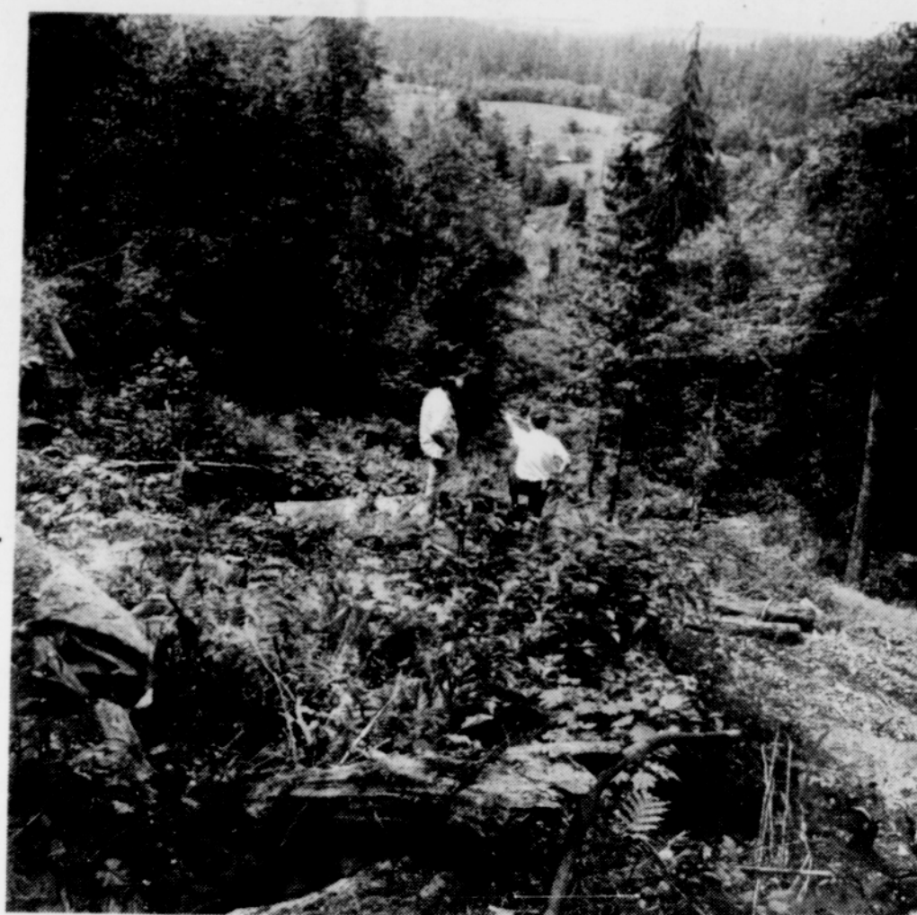
CITY COUNCILMAN James Duff, left, checks out where the improved water line will run along with city superintendent Ken Burdick. The new line which will be in-
