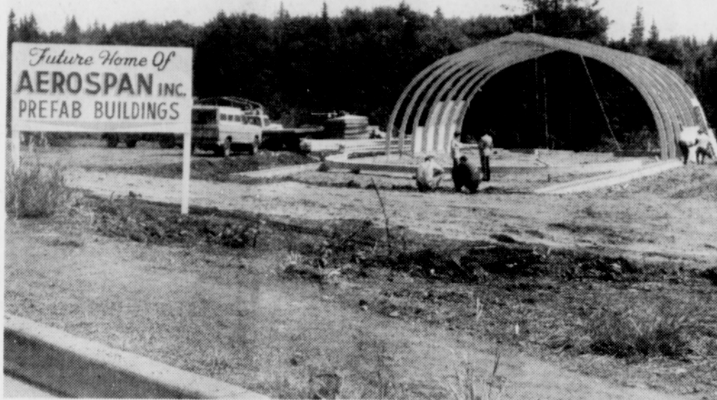
THE NEW AEROSPAN building going up on Main St. is set for completion sometime this month. The firm is planning to move
