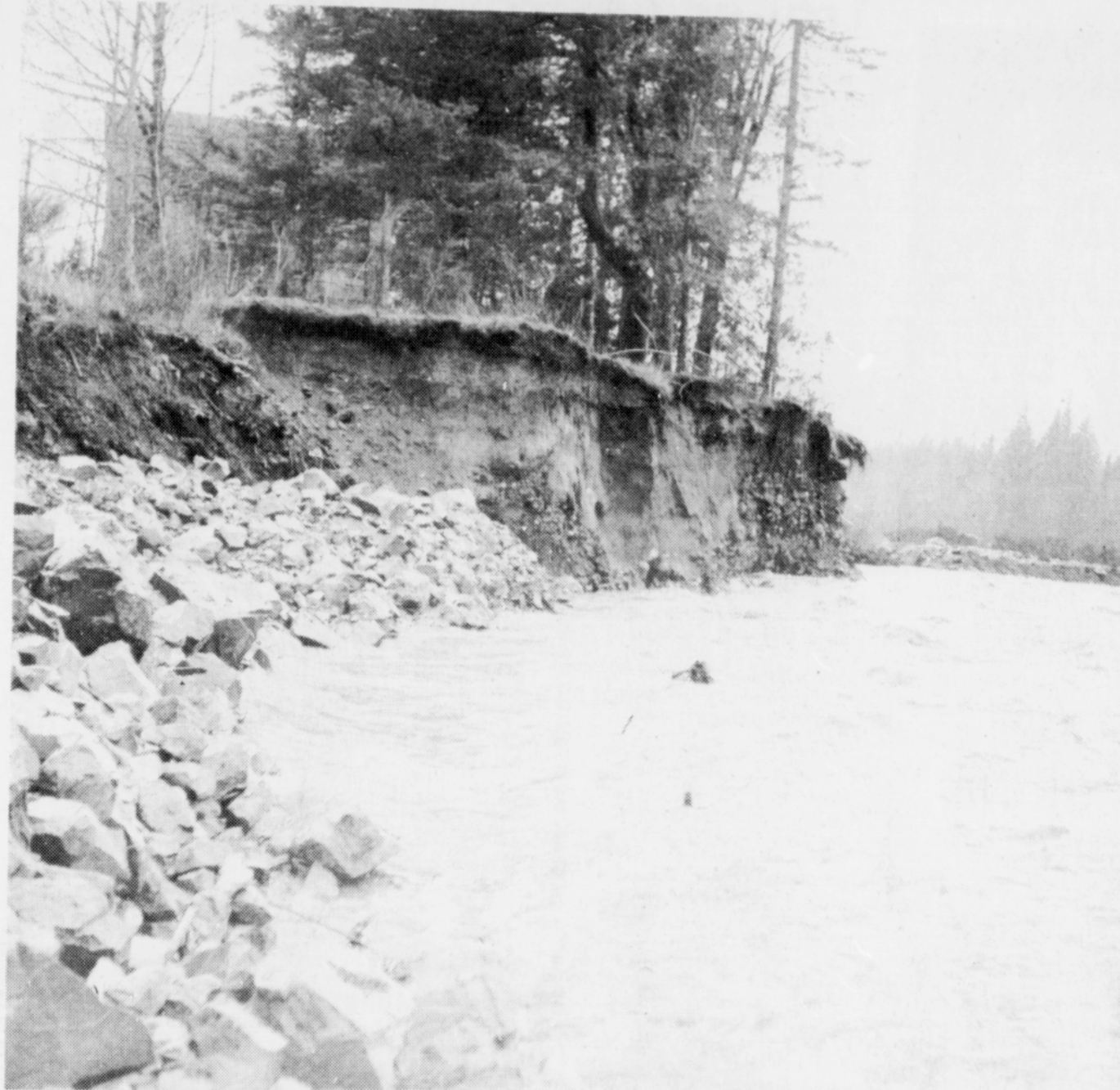
WATERS IN THE Sandy River like other streams in the area were on the rise during the past week. Here at this section of the river near Wildcat Creek along Highway 26 the river can be seen cutting the bank away under Chuck Conarty's home which is located on the ground to the left in the picture. Conarty said he has been fighting the state
