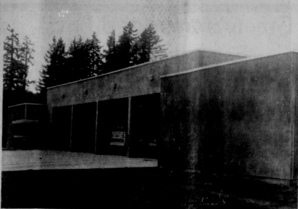
BORING FIRE District has now moved to this new station east of town. The new $200,000 facility is modern in every respect. Surprisingly the cost added only .3 cents per $1,000 property value to the tax roll. (Outlook photo)
