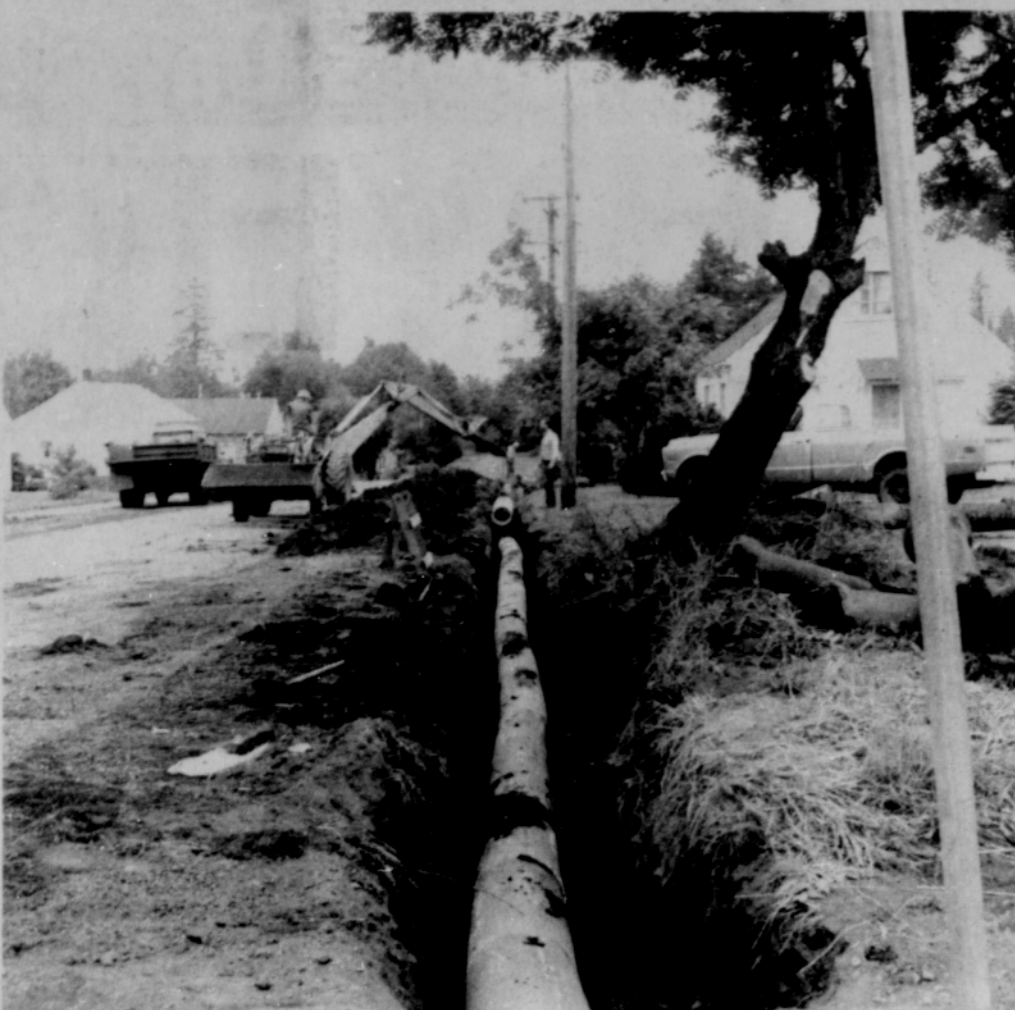
NEW STORM SEWER RUNNING north on Center St. was in process of being installed this week. Work on project is expected to be completed next week. (post photo)
