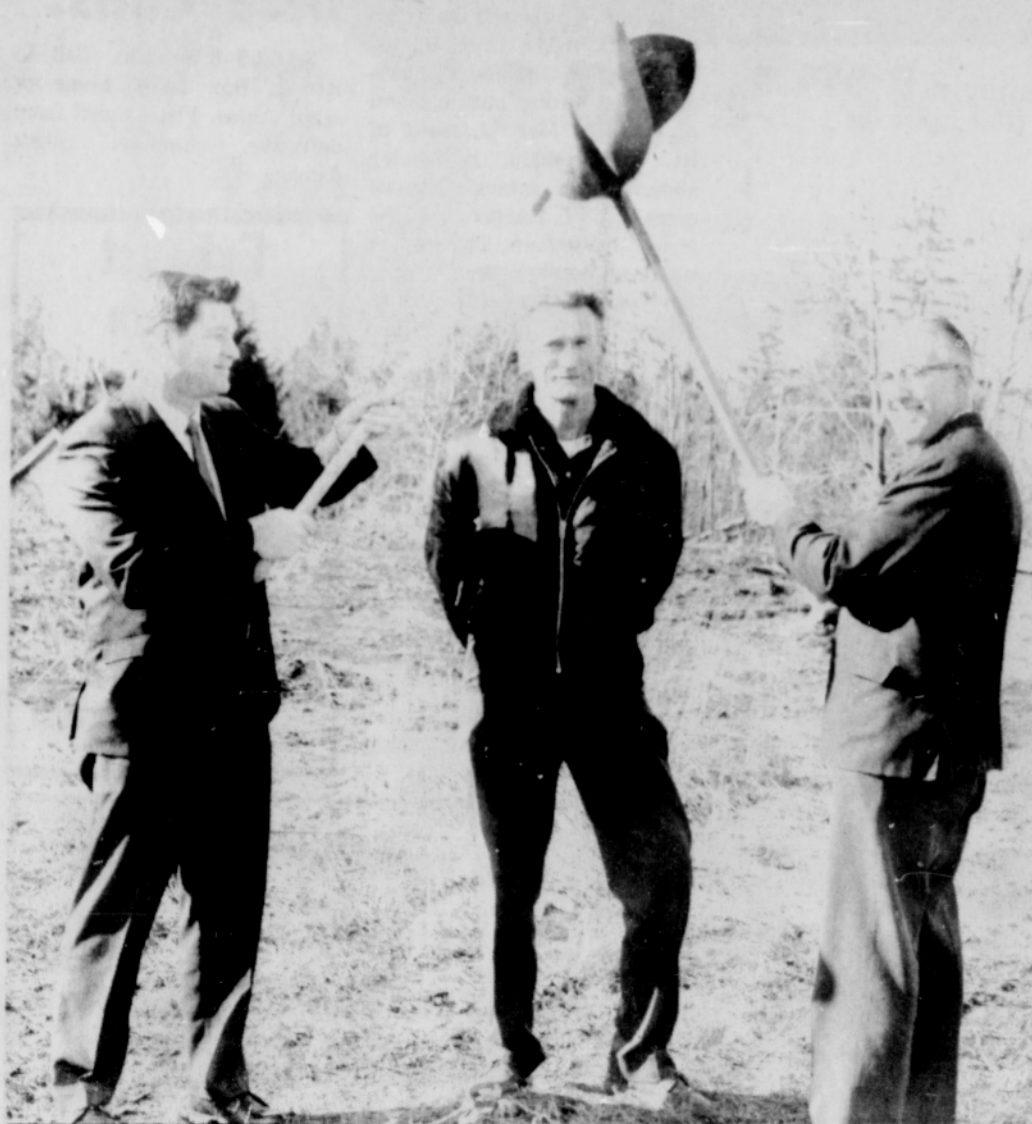
UNOFFICIAL GROUND BREAKING ritual for Sandy's new city hall was held Monday morning when Olin Bignall, right, Chamber of Commerce president and Sandy Kiwanis president George Morgan flourished shovels over head of Mayor Harold Edes in celebration of start of work on site preparation. Building is due for completion this fall. More dignified, official public ceremony is scheduled for cornerstone laying early in April. (Post photo)
