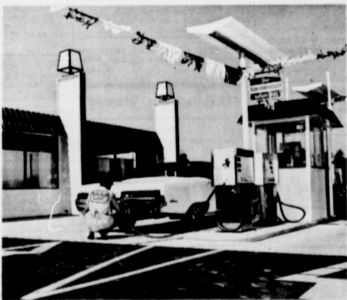
1—Simply drive into either one of our two new modern Gresham RUB-A-DUB MINI WASH Gas Stations and say, "Fill 'er up!"
