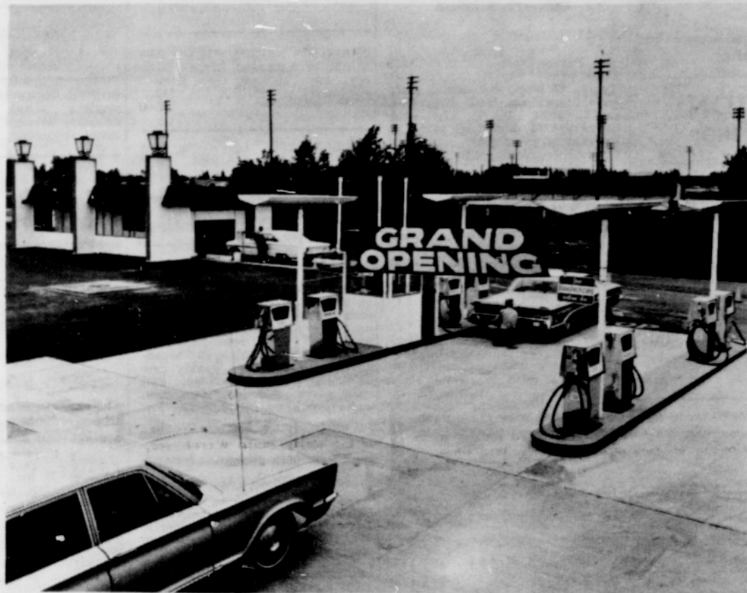
Burnside Extension (1/2 blk. East of Main Ave.)
