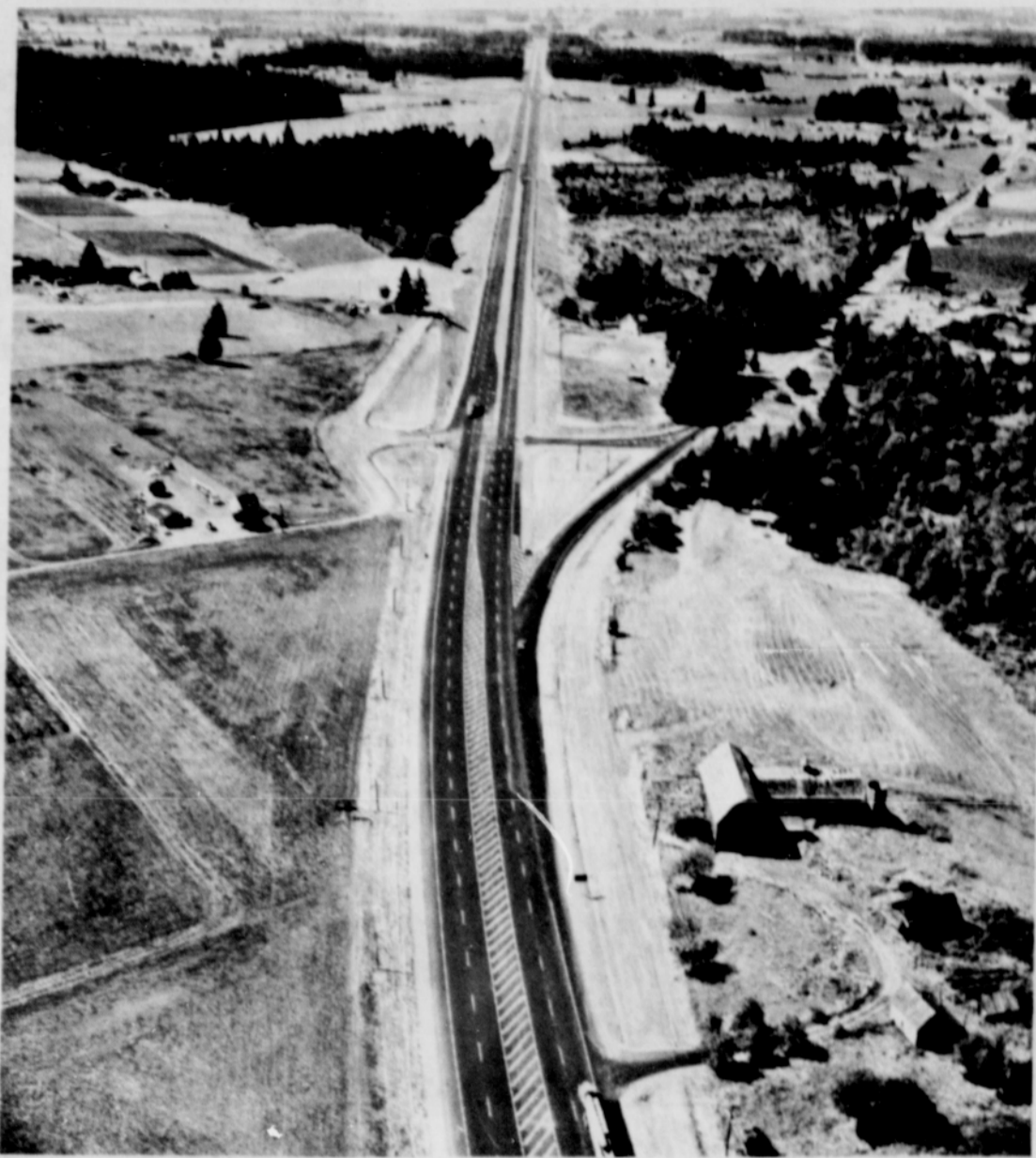
One of the major projects completed by the Oregon State Highway Dept. this year was the new Mt. Hood Loop Highway. Shown here is the new section looking westerly from Sandy, Old Highway angles off to the right. The 8.25 miles of the new road was completed in July at a cost of $2,190,925. (Oregon State Highway Dept. photo)
