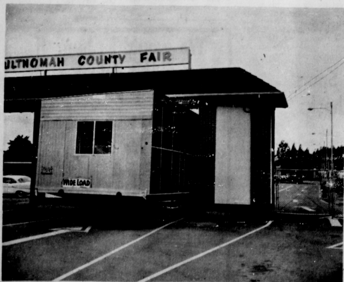
It was a tight squeeze for this portable trailer classroom to pass through the gate at the county fairgrounds in Gresham. Classrooms were delivered in half-sections and then assembled at the fairgrounds into 24 by 57 feet classrooms for Mt. Hood Community College which starts sessions Sept. 19. Trailers were made in Vancouver, Wash.
