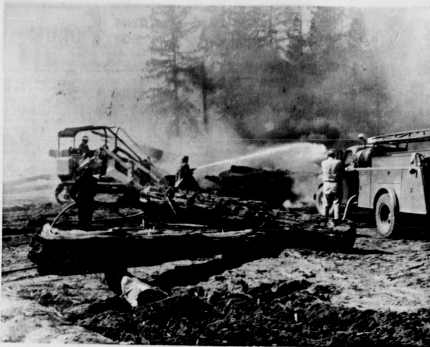
MEN AND EQUIPMENT battle blaze at Alder Creek box factory. Here dozer pulls logs from cold deck while firemen pour water onto blazing logs. Lack of nearby water supply hampered fire fighters as tank trucks ran dry.
