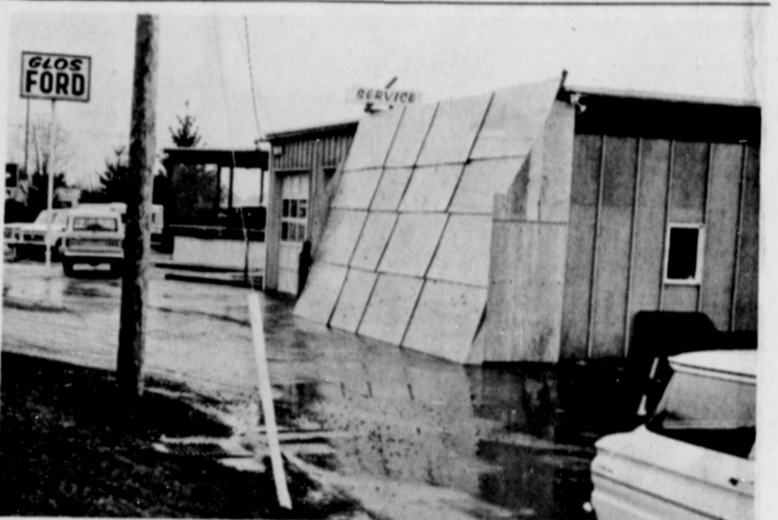
GLOS FORD AGENCY shop in Sandy sustained $2000 damages when small Datsun pickup crashed into building late Friday night. Young driver fell asleep at wheel. Car was damaged extensively, driver was hospitalized with severe head cuts.
