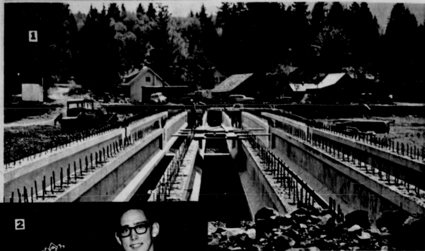
Picture events of May: 1. Seven pre-stress concrete girders were set in place on the Brightwood Bridge project by the county as the bridge is taking shape again. It was under construction when the Christmas floods struck the area badly damaging work already completed. 2. Crowned as "Queen of the Jr.-Sr. Prom" at Sandy High School was Connie Schwendemann. She is shown with her escort for the evening Bob Fredrickson. 3. Looking at his strawberry field near the Mt. View Golf Course in Boring is Don Eckland. The field is in full bloom.
