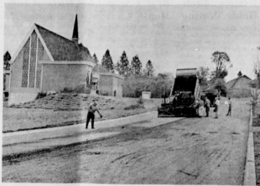
It's a new paved street for Sandy. Here workmen put down asphalt paving on East Pleasant Avenue. At left in the picture is the Immanuel Lutheran Church.
