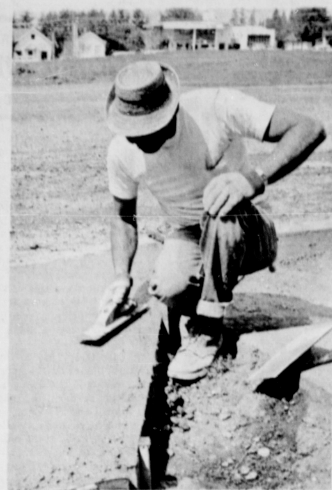
Putting on the final touches to the sidewalk with hand trowel is this fellow. Street is progressing rapidly along the Main Street. (Post Photo)
