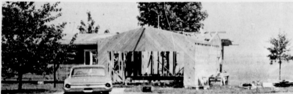
This addition being built just east of the Sandy city limits on the Loop highway will include one additional room and a double garage. The home belongs to Woodrow W. Carter of Sandy. From the backside of the building a beautiful view of the valley below, Mt. Hood, Roslyn Lake, and Rich's Airport are available to the viewer. (Post Photo)
