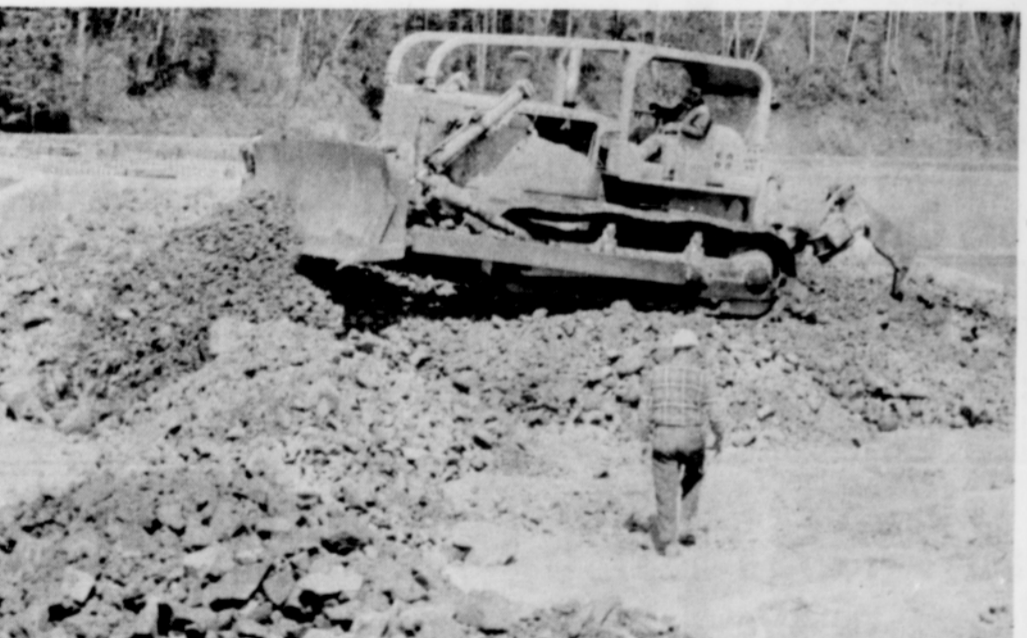
Building up the approach to the Brightwood Bridge is this cat. When the bridge is completed it will provide a roadway from Loop Highway down Brightwood Road and across the Sandy River to homes in that vicinity. (Post Photo)
