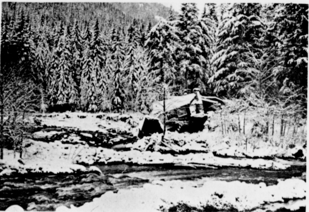
Shortly after this picture was taken the home split down the middle and into two separate sections. It is located to the right of the ZigZag River bridge. Noticeable in the photo are two separate channels of the river, whereas only one channel existed prior to the recent flood.
