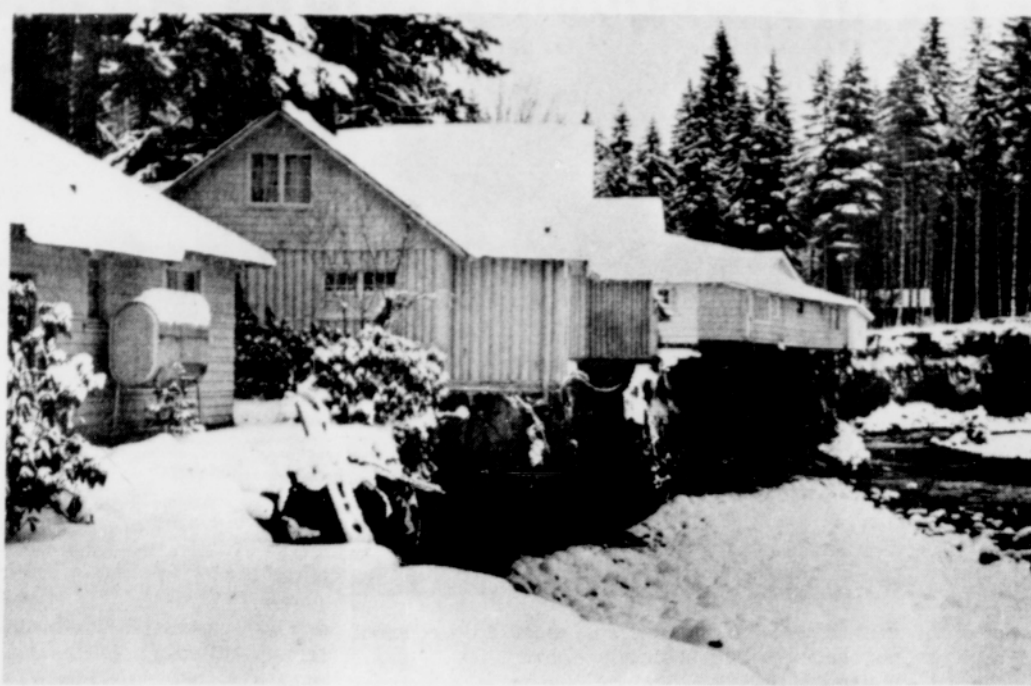
Resting in midair are the latter portions of these four homes located behind Log Lodge. The earthen foundations have been washed away by flood waters. Progress towards moving these homes to safer ground is now under way. In fact, the fourth home from the left has been moved.
