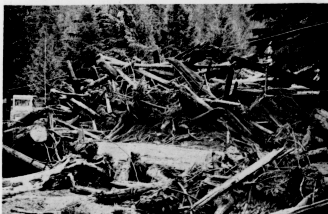
This pile of wood, logs, stumps, houses blocked US 26 at Wildcat, caused water backup as cut-over land flooded in last week's rains, snow melt. Picture shows highway in center. Height can be measured by road grader.
