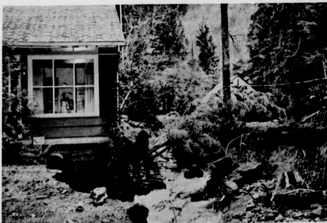
Creek took new course, undercutting home shown at left. This was taken two days after flood.
