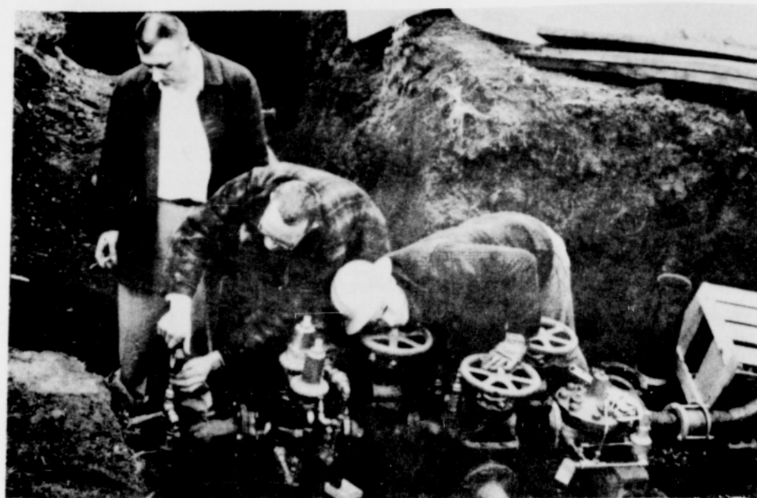
Mayor Paluck, Russel Shaver and Lew Isenburgh test the new by-pass for the Sandy water system. It worked perfectly and will allow the tank to be drained for cleaning and needed repairs. Without this by-pass the city would have been without water during the repair time estimated to be about three weeks, an impossible situation.
