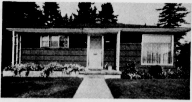
"We wouldn't have any other type of heating," says Mrs. Richard Talmage, 7319 S. E. Center Street in Portland. "Our ceiling cable heat keeps our 962 square foot home warm as toast."
