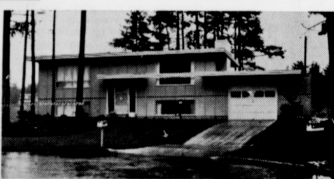
"Electric heat has been very economical and trouble-free. We love it," say the Jason Evensens, 17435 N. E. Flanders in Portland. Ceiling cable heats 1824 sq. ft. Insulated ceiling and walls.
