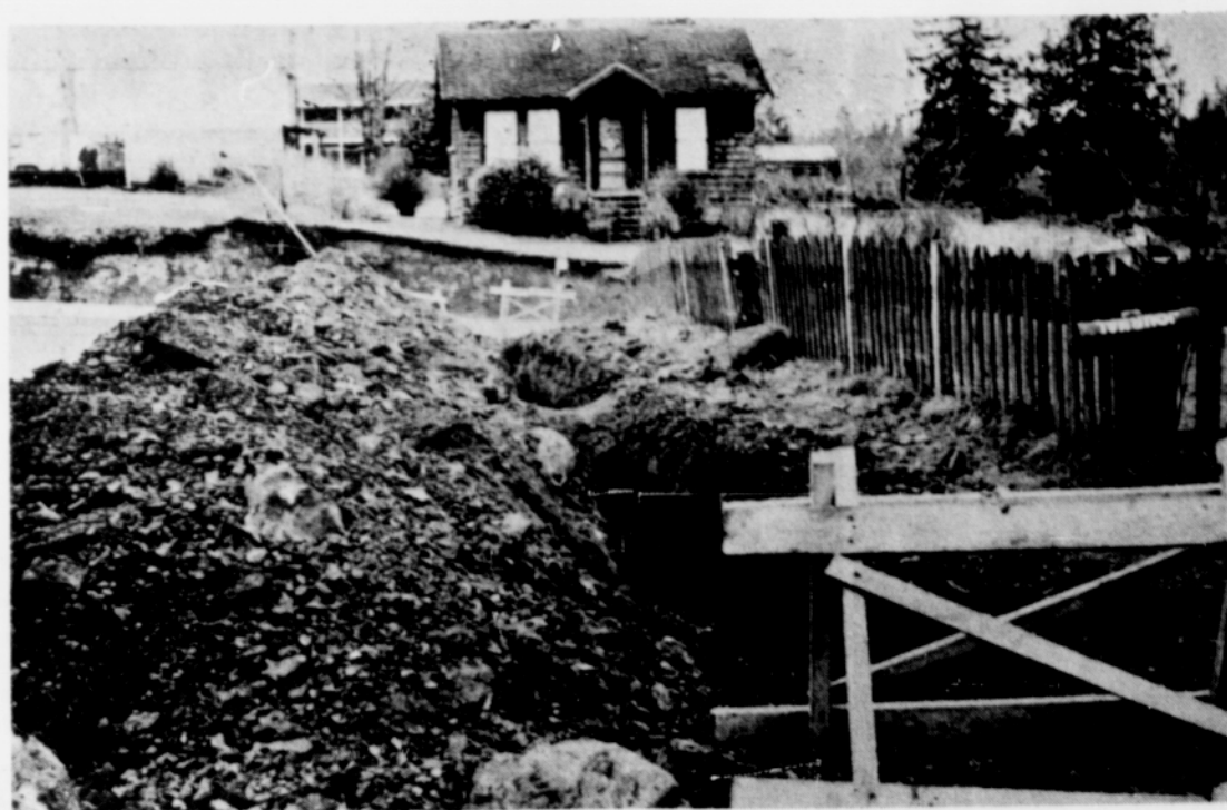
Excavation work is being done on Sunset St. preparatory to laying new six-inch water pipes to replace old line. The new pipes will hook into the four-inch line on Bluff Road. Final hook-up will not be made however, until the voters make a final decision on water meter installation. (Sandy Post photo)
