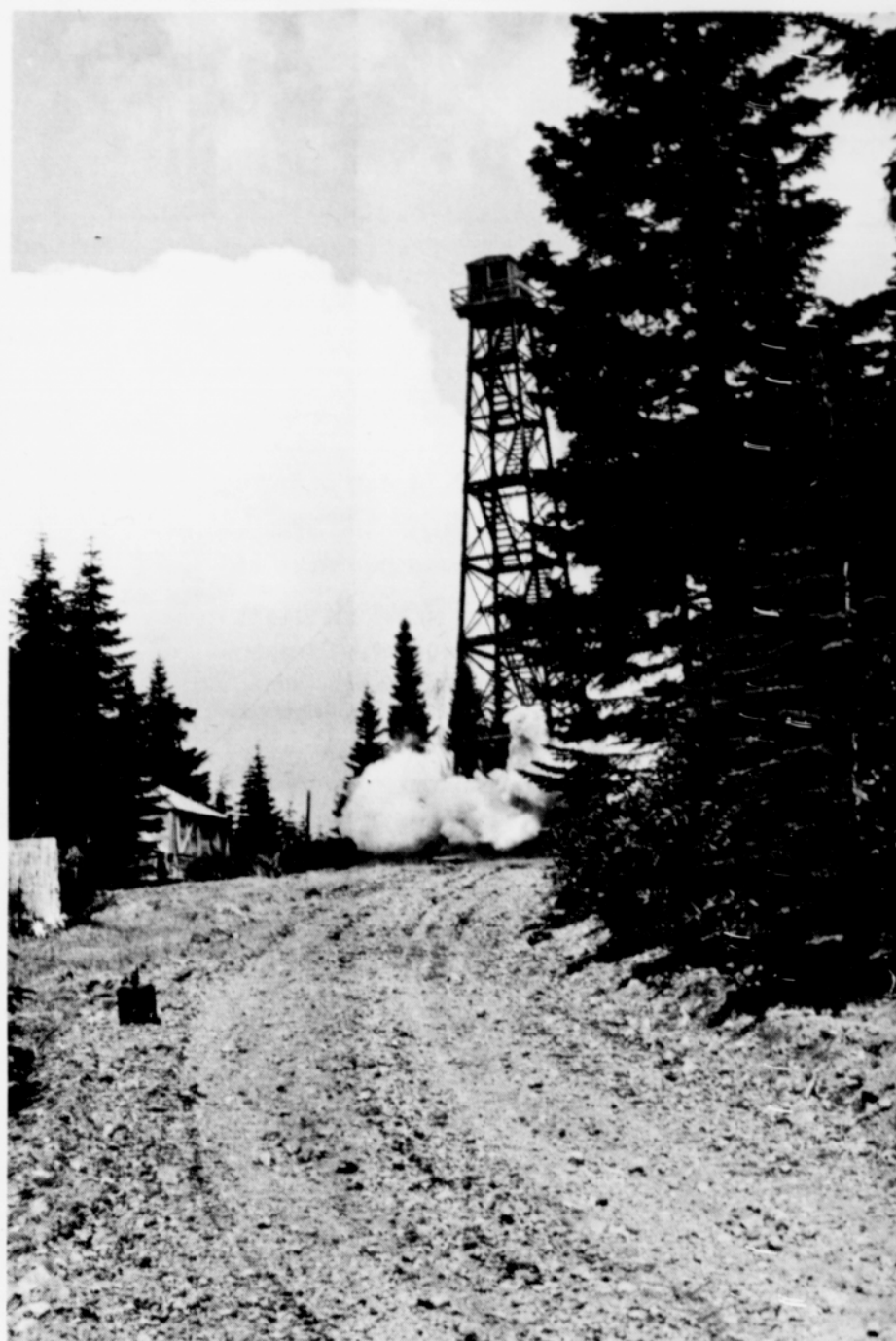
The old lookout at Aschoff Butte on the edge of the Bull Run Watershed came crashing down to make way for a helispot. Forest Service men dynamited one leg of the old structure
