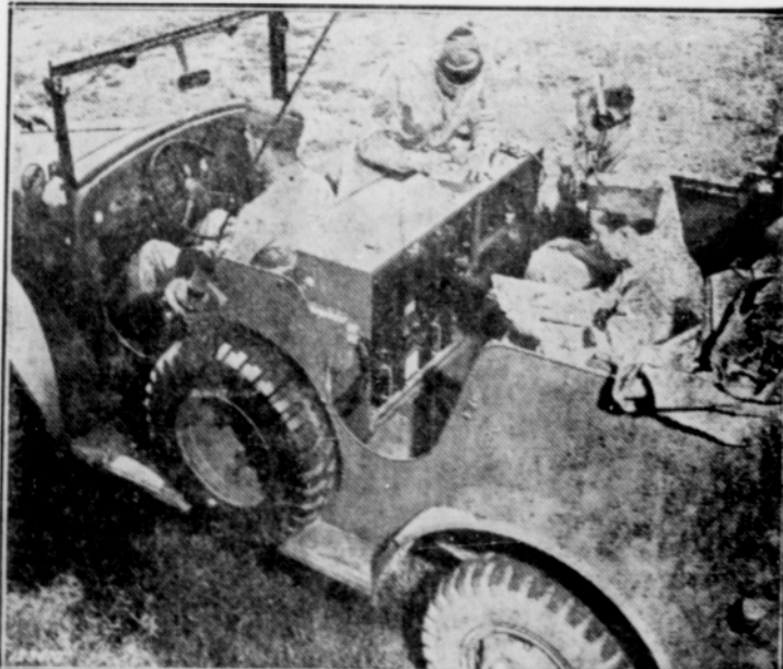
Signal Corps Truck Switchboard
