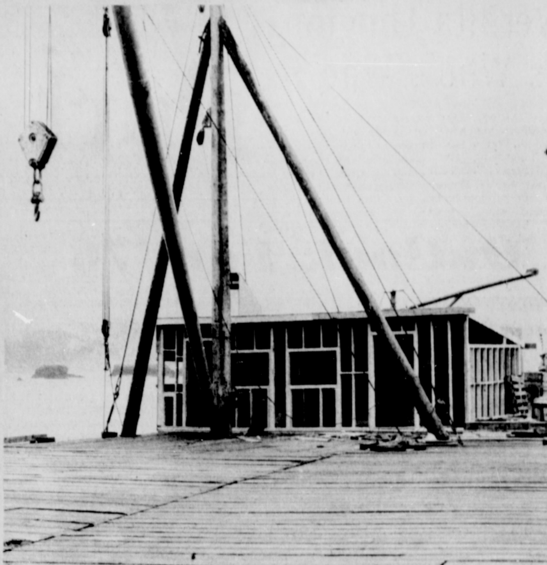
WITH COMPLETION of the re-decking project under the boat hoist, efforts are being directed to finishing a combined hoist engine housing and harbormaster's office at the commercial dock. Emergency dredging alongside the dock under the boat hoist area is also scheduled to begin in the immediate future with a dragline dredge on loan from the Port of Gold Beach.
