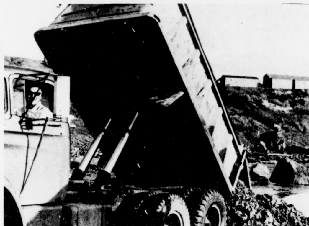
ROCK TRUCKS were moving again this week as contractor nears completion of new parking areas at local port. Truck is unloading rock here between cannery and dock approach.
