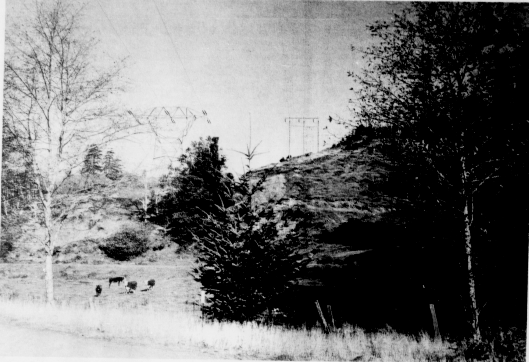
Bonneville Power Administration's Bandon-Gold Beach 115,000-volt Lines No. 1 (r) and No. 2 (l), near Sixes, Oregon.
