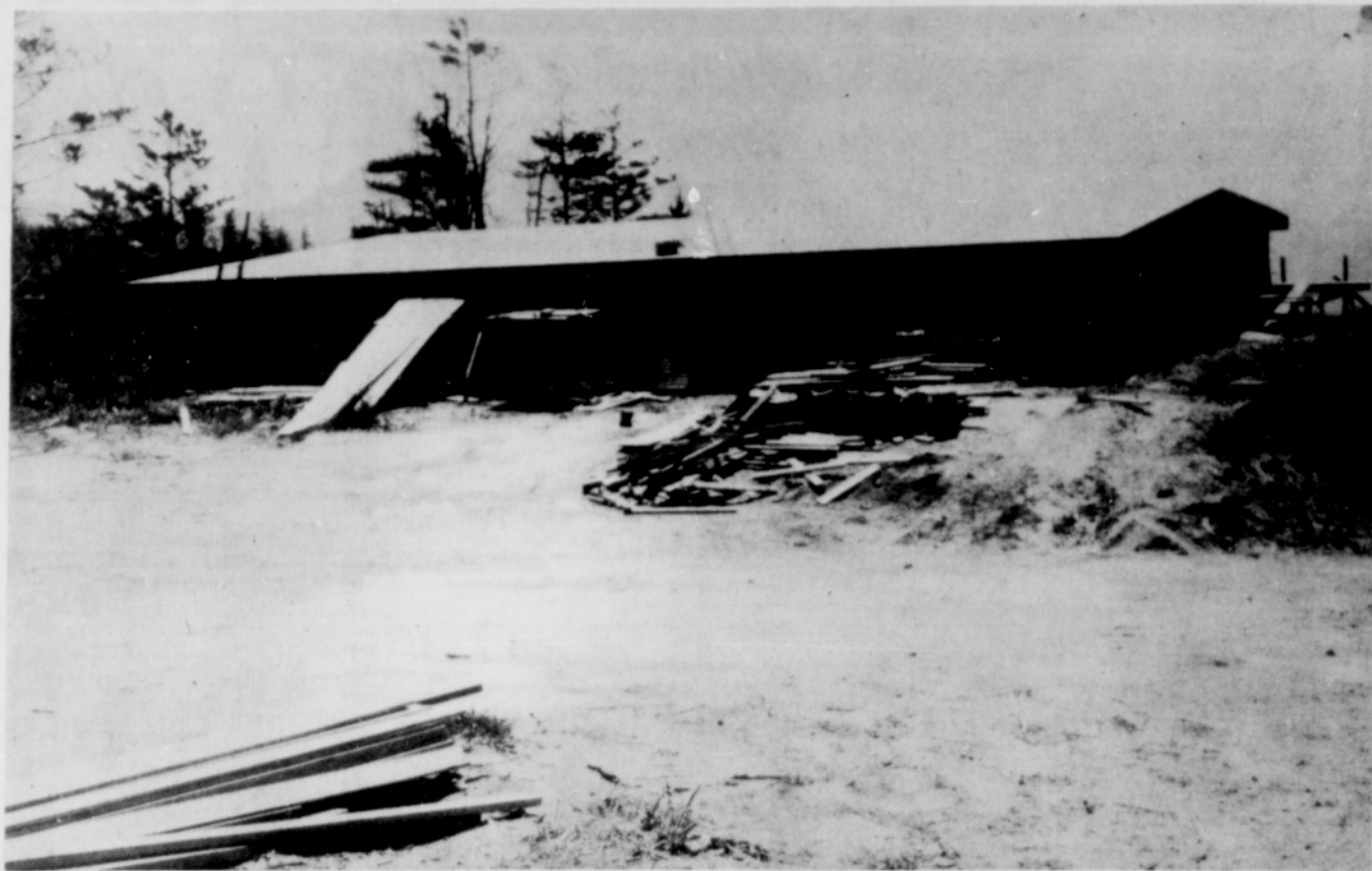
THE NEW city water reservoir cover was nearly ready for roofing Wednesday as crews finished laying plywood panels.
