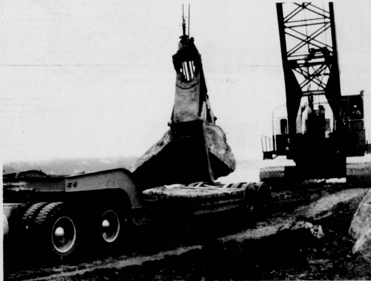
AFTER weighing, trucks are turned around and backed up to huge crane for unloading... then back to the quarry for more rock. Only one rock, of seven-tons, was rejected for the project Monday. 112, 000-tons of rock will be used in the breakwater.
