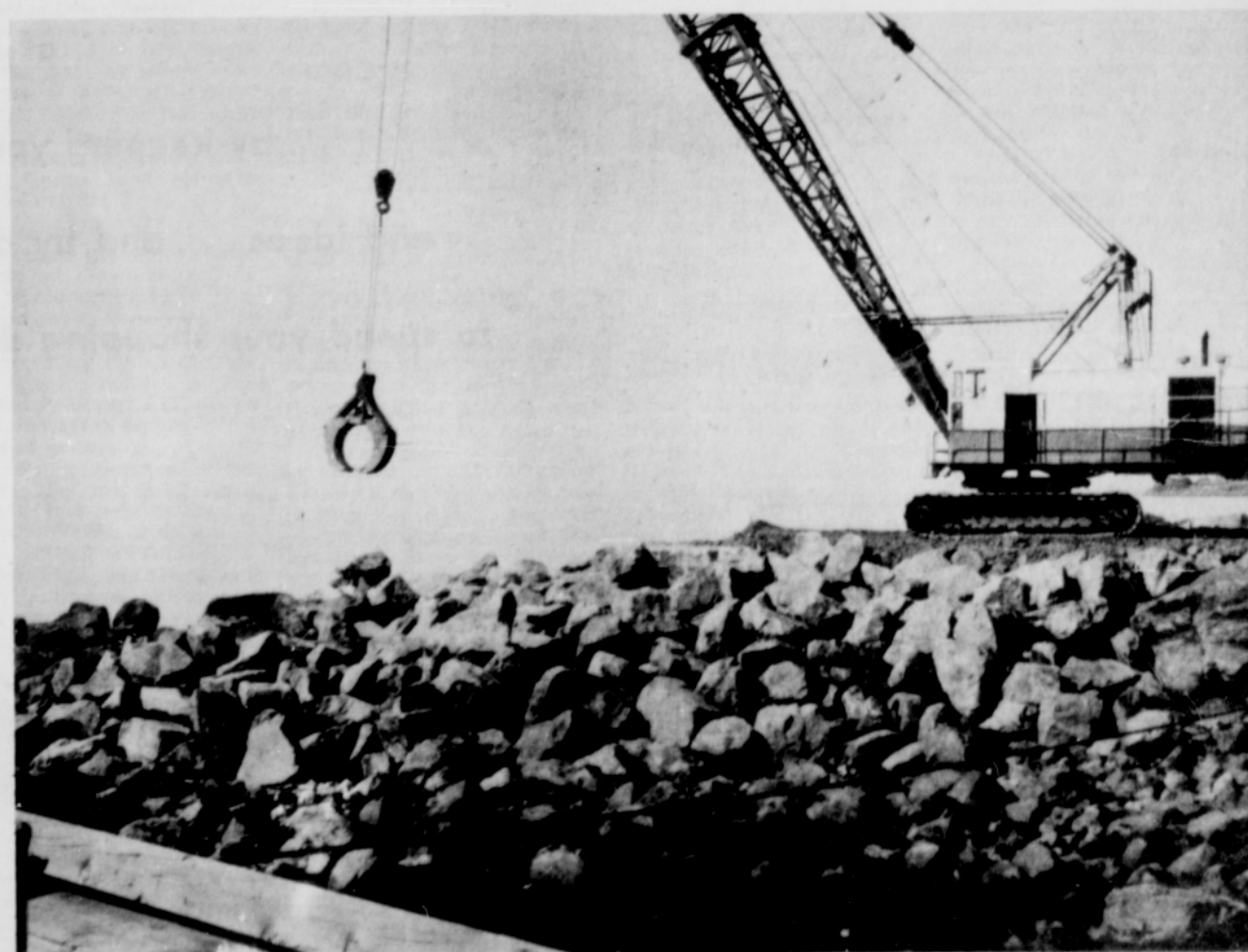
THIS VIEW Wednesday morning from the dock shows amount of rock placed in two days of construction. Roadbed for the Lima crane is built as jetty is extended. Contractor for breakwater is F. L. Somers of Medford.
