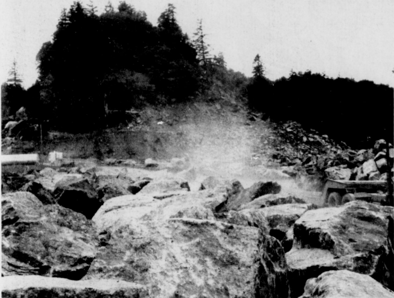
JETTY ROCK starts 10-mile trip to site from quarry up Sixes River on Ryce Wilson ranch. Hill in background is nearly solid rock. Huge rock in foreground are stockpiled for loading. Quarry work started the last of April.
