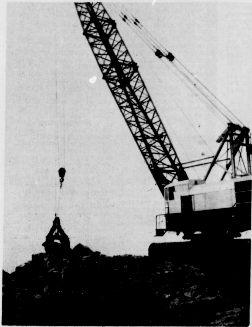
VIEW from breakwater area shows first rock being placed Monday morning.
