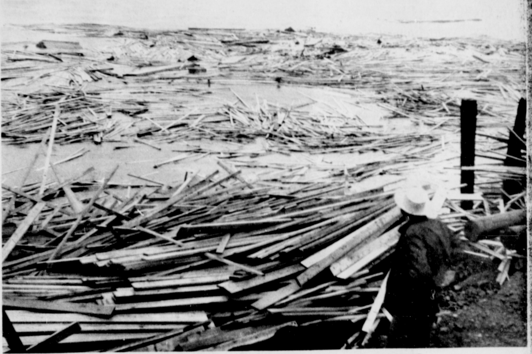
THE DATE: February 1959. This shows part of a million feet of lumber lost when a storm took out the dock. This damage, and subsequent losses could have been prevented by a breakerwater.
