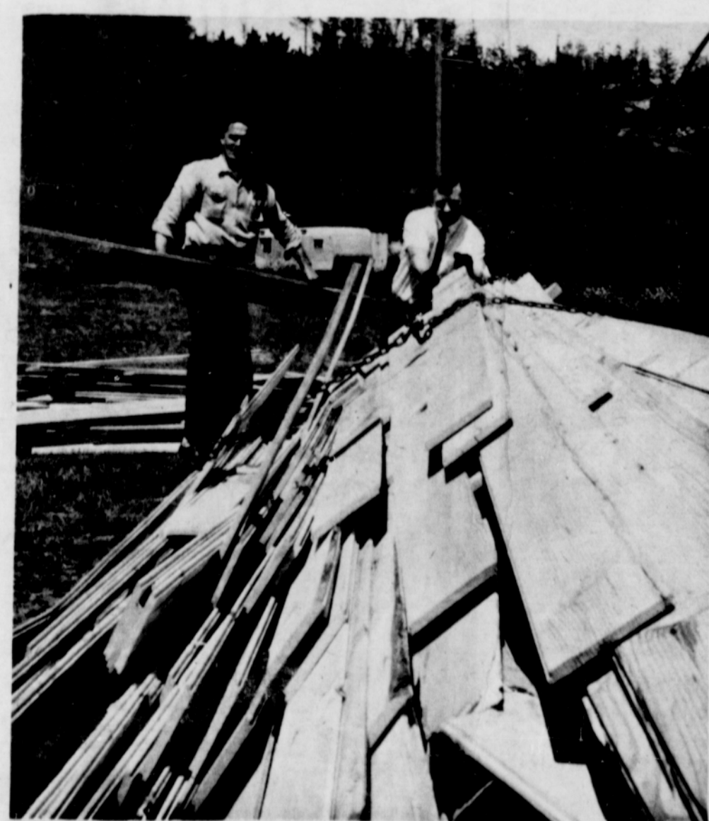
JAYCEES Jiggs King and Jim Peterson, club president, are getting an early start on construction of the Indian Village, an outstanding feature of the July 4th Celebration. This load of lumber was dropped at the site, opposite Battle Rock State Park, last week. Construction of the corral-type enclosure will start this week.
