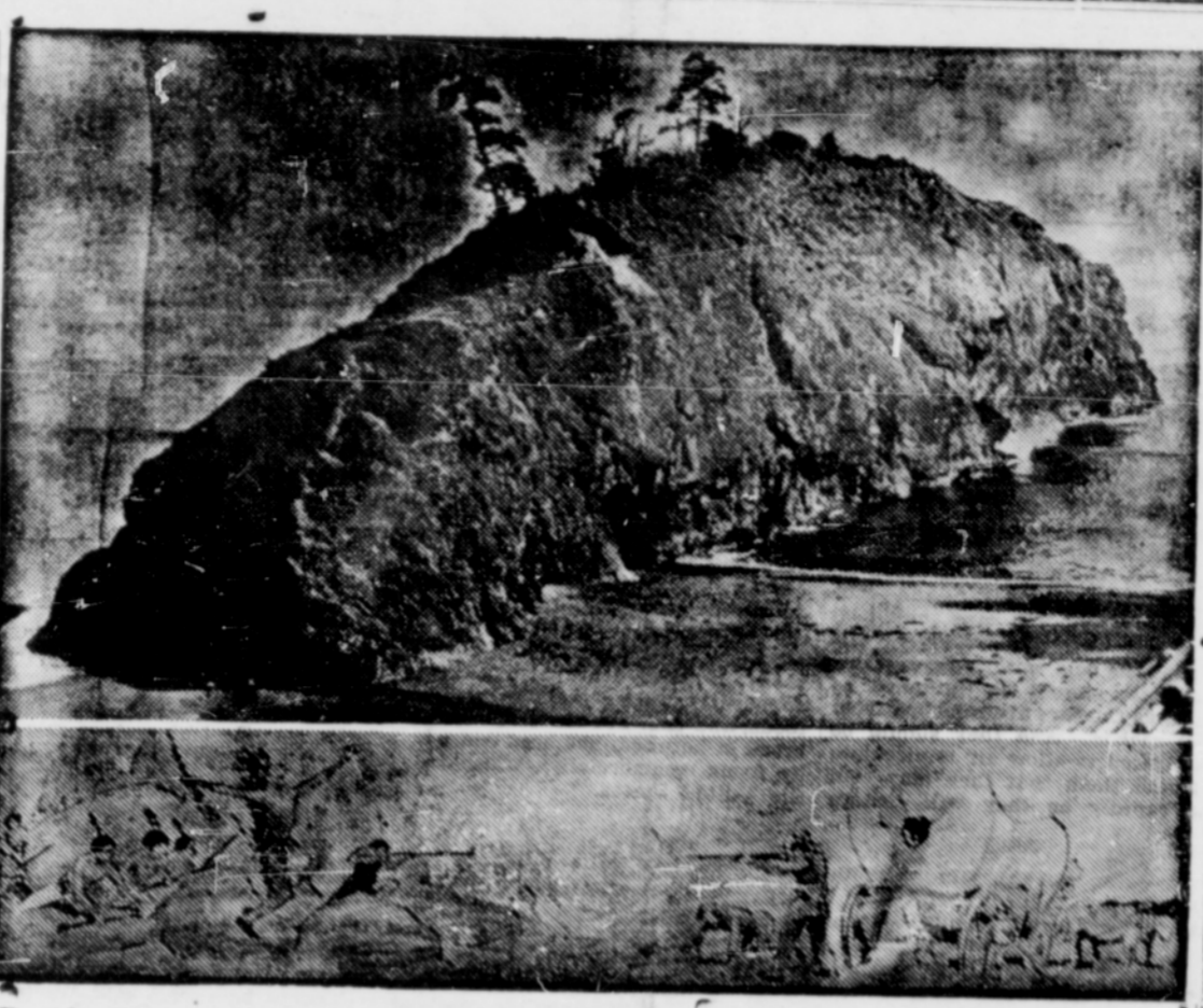
Battle Rock, Port Orford landmark that is one of the points of interest along the Oregon Coast Highway.
