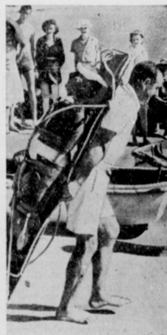
This new type of stretcher, invented by an Australian, is being demonstrated on the beach at Sydney, Australia. It is designed for use in bombed buildings by one-man rescue expeditions. The stretcher's straps and footrest will hold a patient firmly, even when tilted at a sharp angle as shown here.
