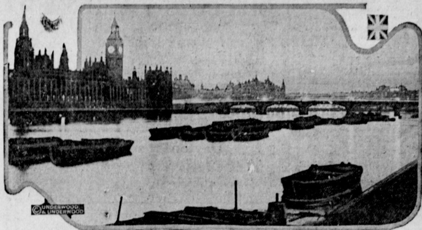
Here is a most remarkable view of the Thames at night, taken during the recent heat wave, when the atmosphere of the usually foggy city was startlingly clear. On the left bank are the houses of parliament.
