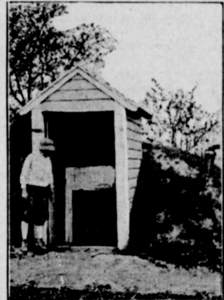
An Outdoor Storage Cellar, Built Partly Underground, for Storing Garden Vegetables. It Is Built of Concrete Except the Entrance, Which Is Frame, and Is Frost Proof. Where the Cold Is Not Severe Less Protection Than Is Shown Here Is Needed.
