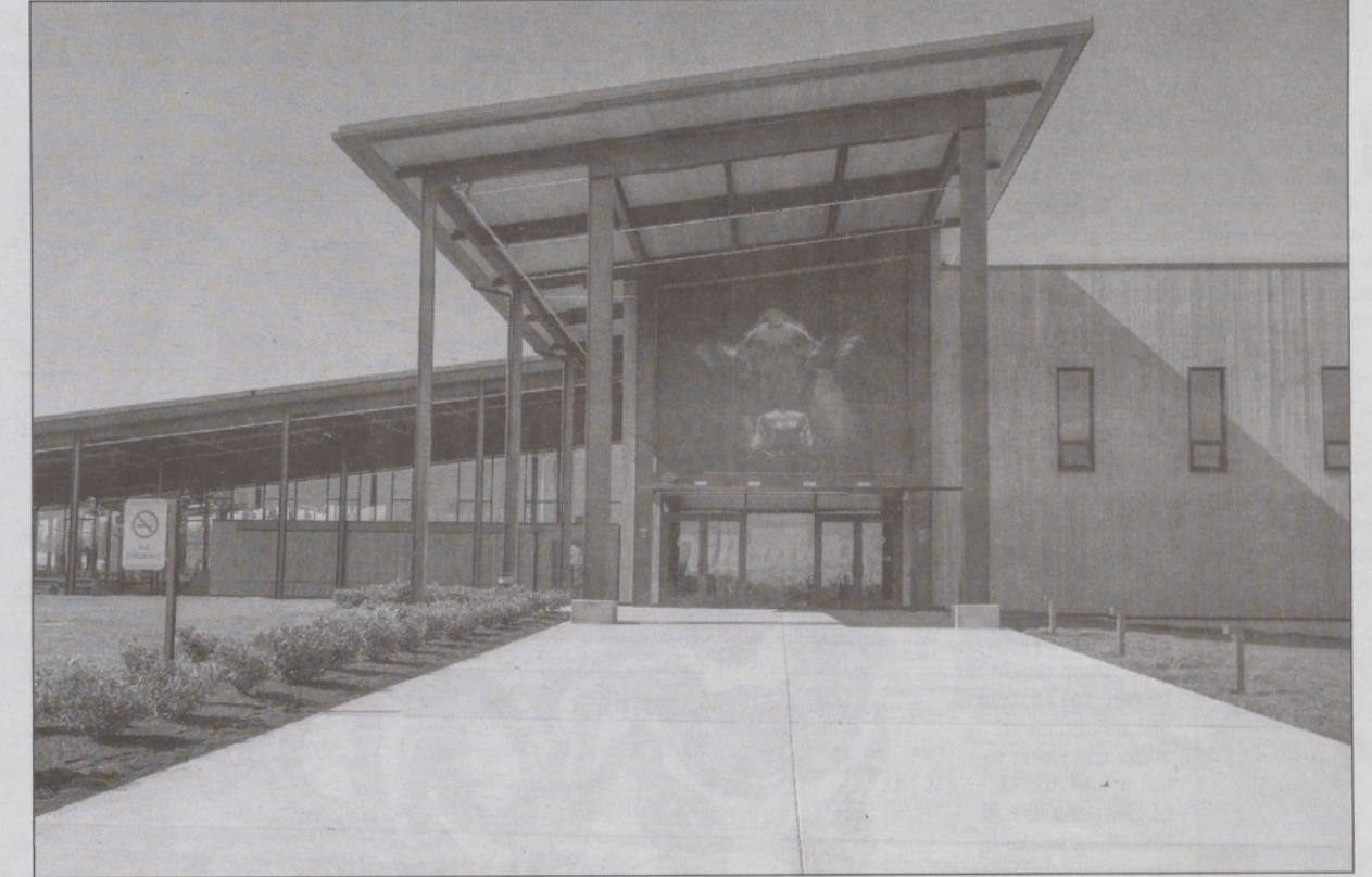
The newly constructed Tillamook Creamery and visitors center.
