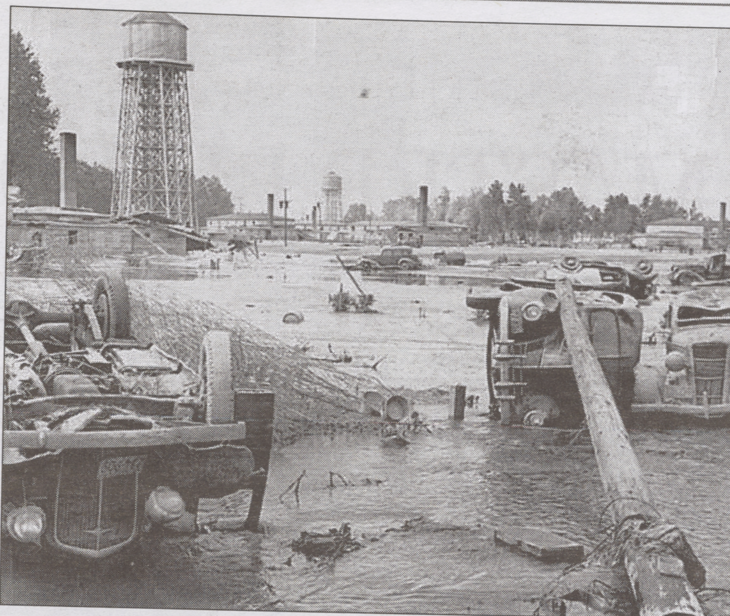
PHOTOS COURTESY OF PORTLAND CITY ARCHIVES Devastation in Vanport after the flood waters receded.
