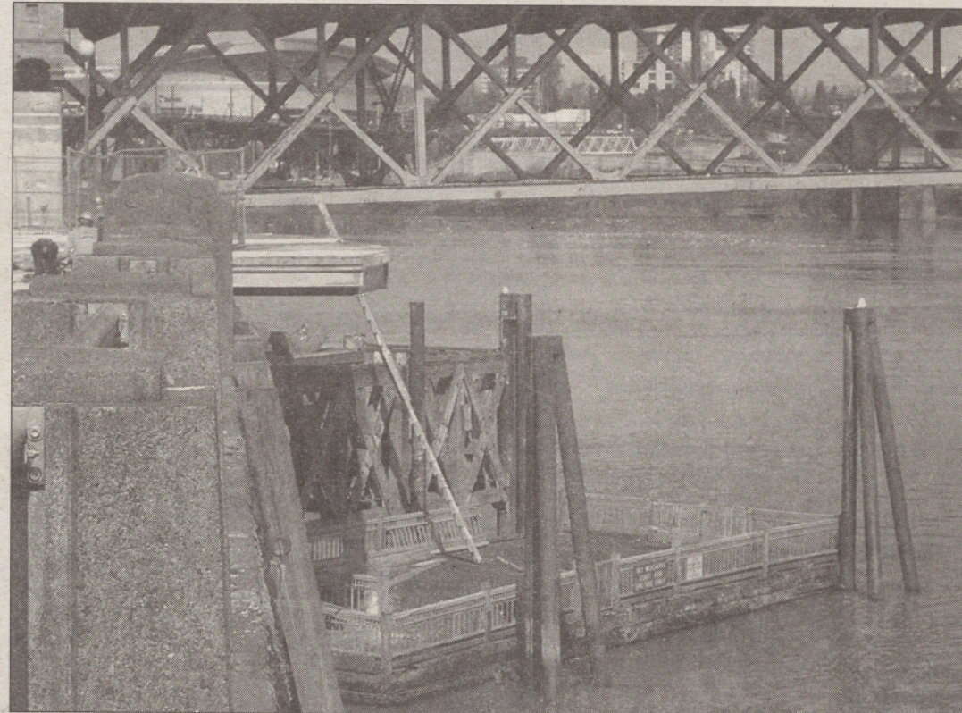
The Murnane Wharf perched off the west bank of the Willamette River.
