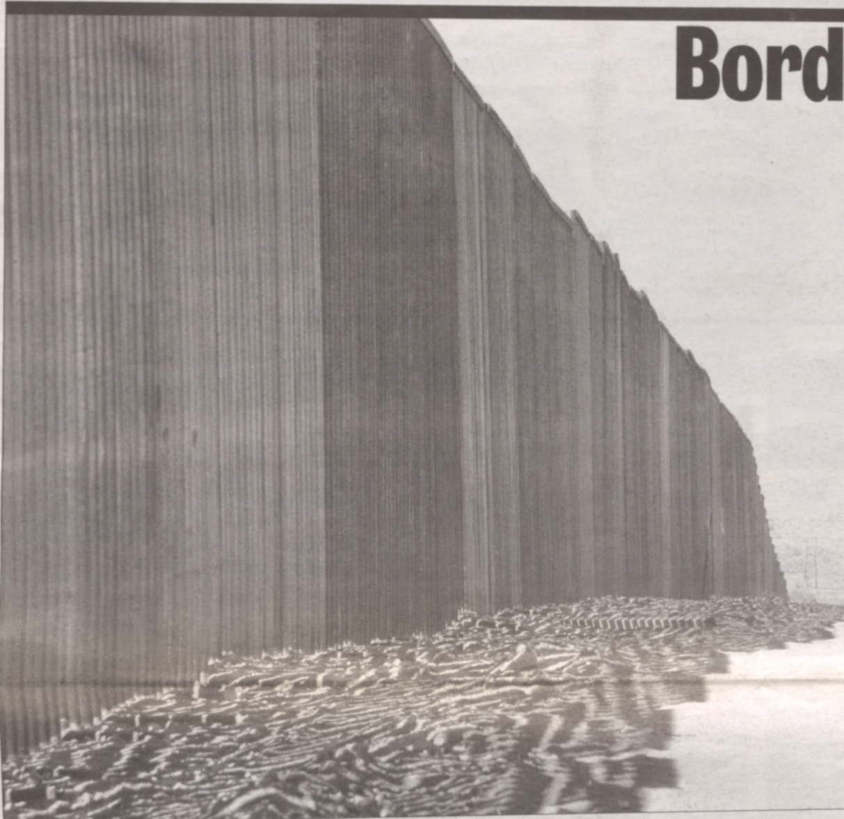
The new border wall between U.S. and Mexico at Sasabe, Sonora.
