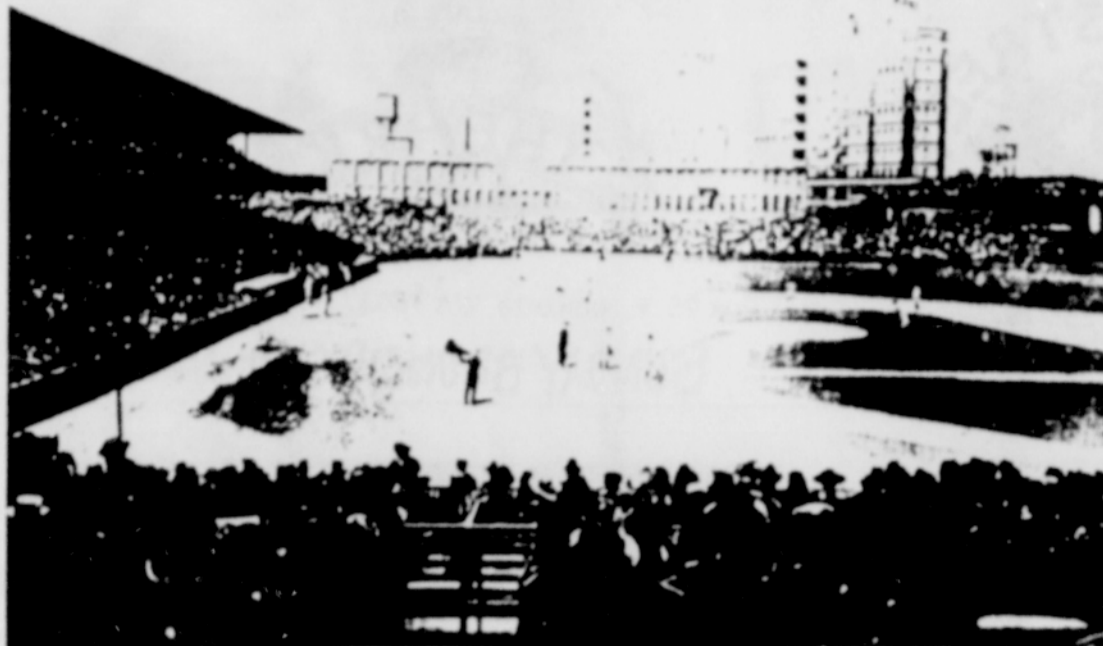
Baker Bowl , Philadelphia - Fatal accidents due to collapsing grandstands occurred here. Twice.
