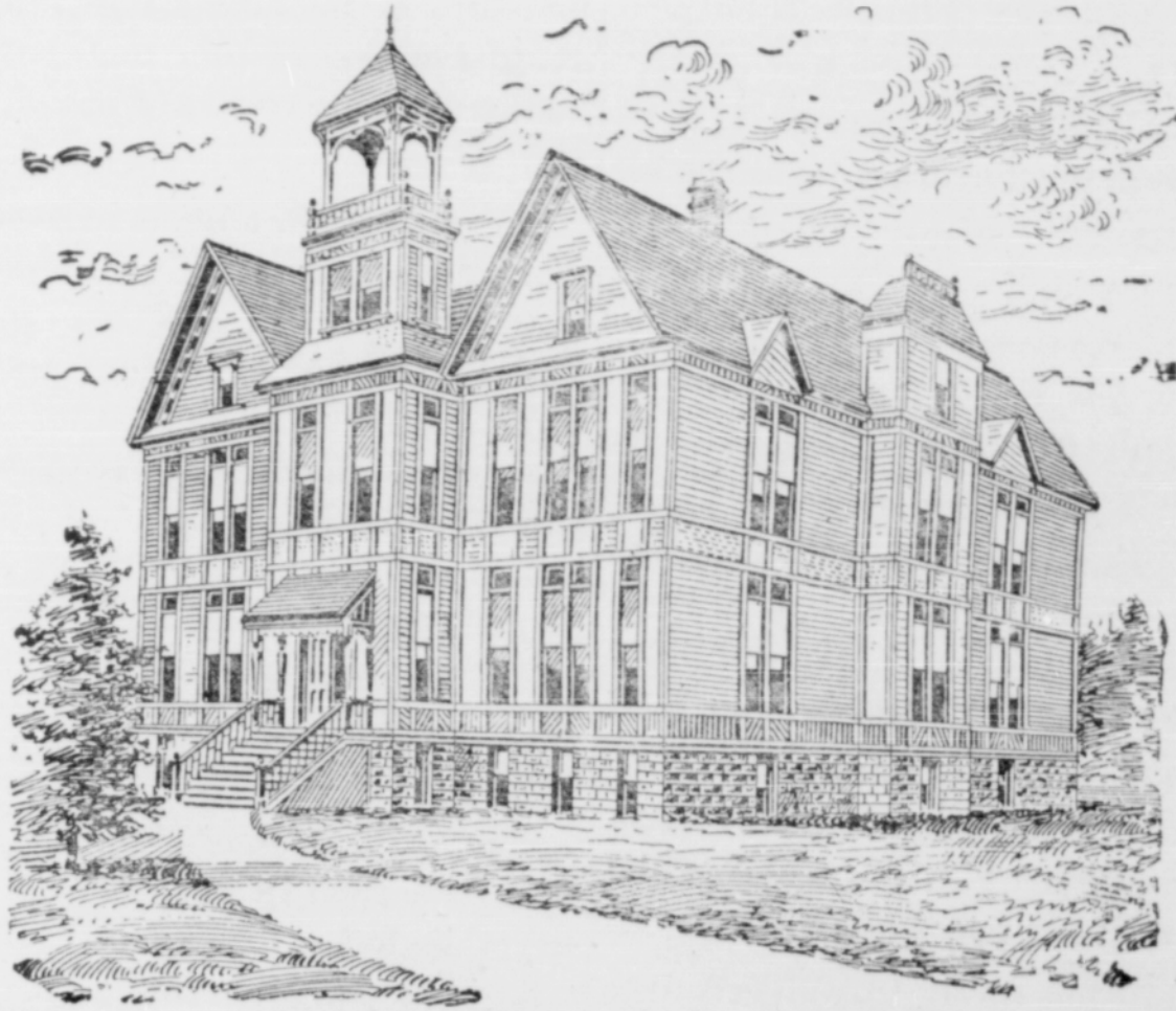
Building in Course of Construction.
