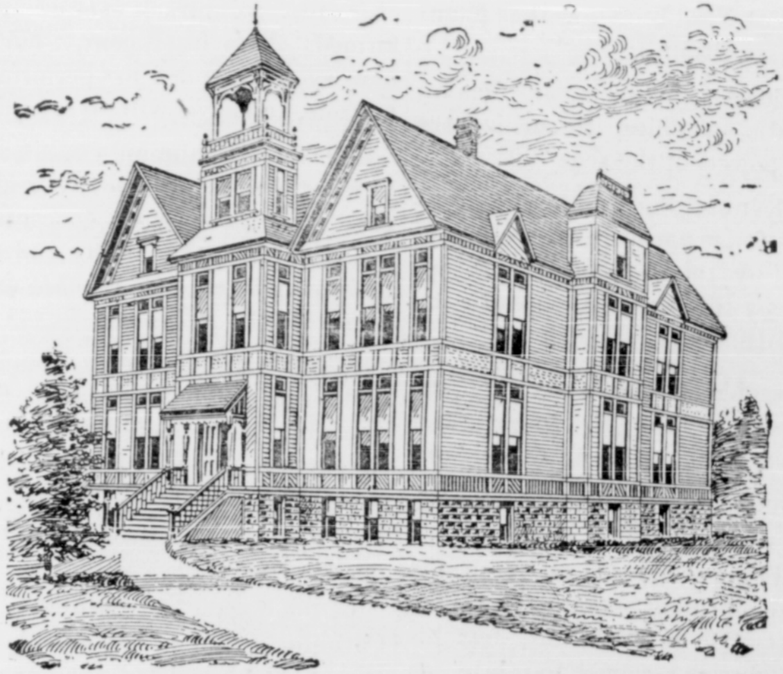
Building in Course of Construction.
