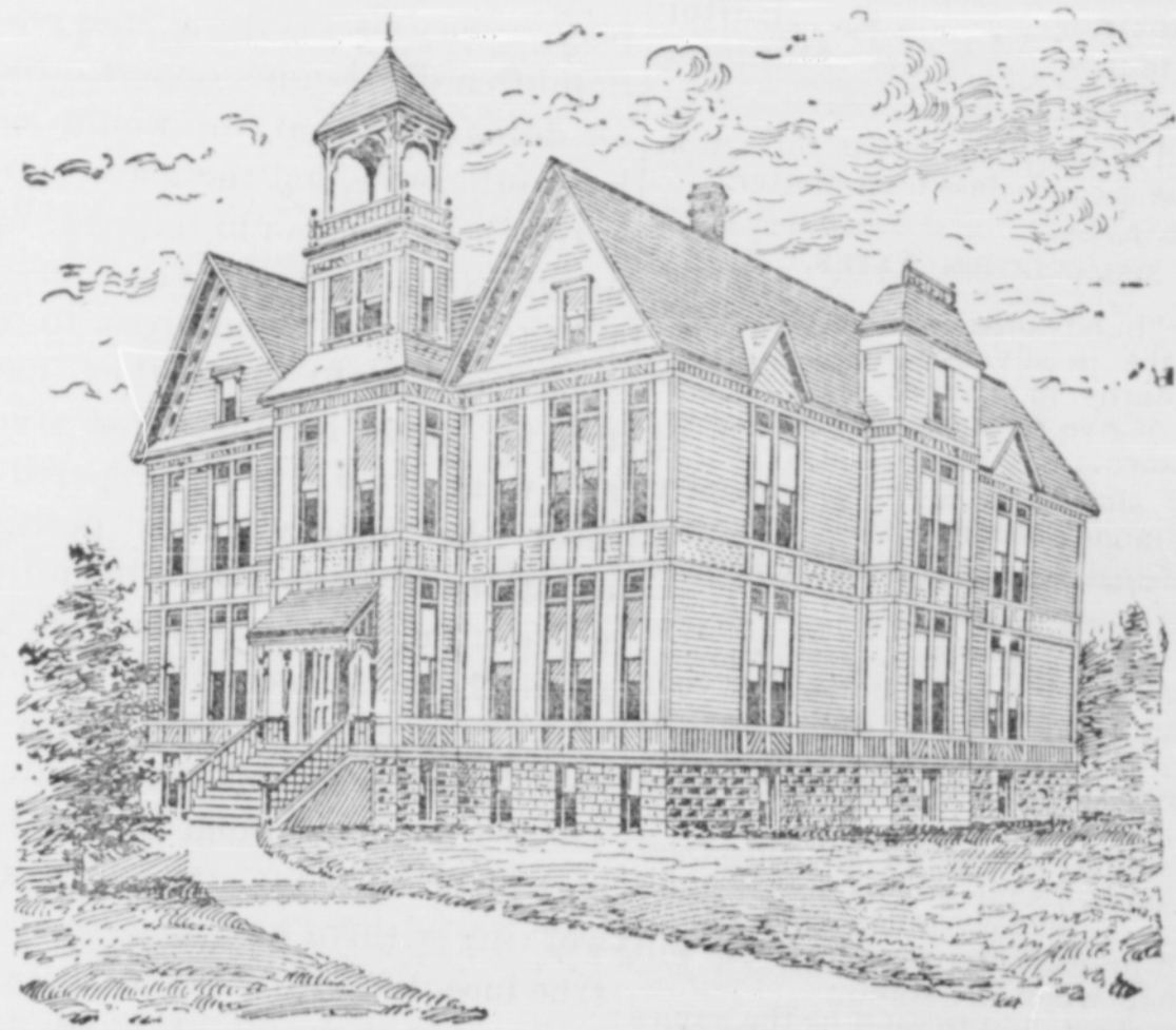
Building in Course of Construction.
